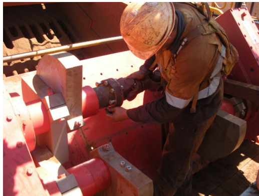
Photo No 30: Inter Gearbox drive shaft being refitted
