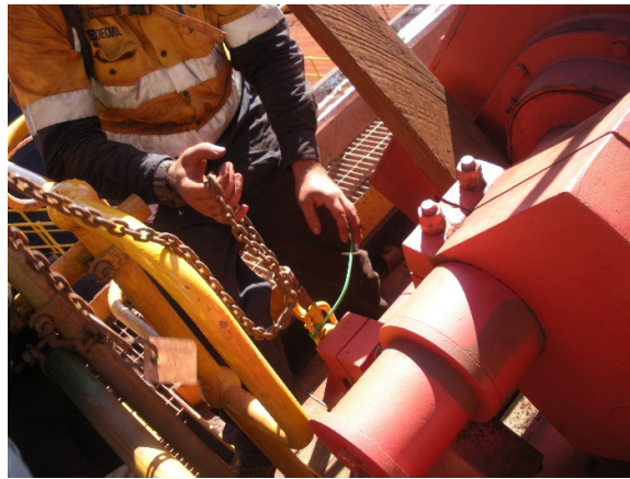
Photo No 21: Lifting attachment fitted to counterweight
