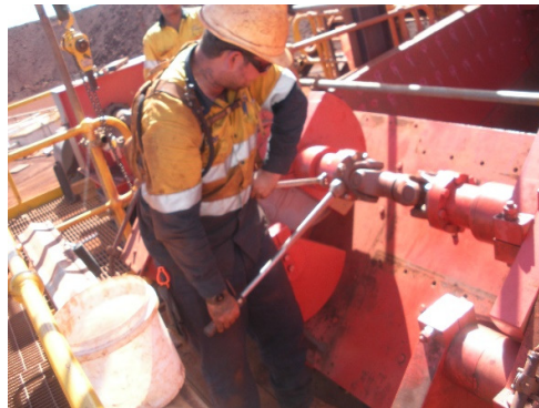
Photo No 32: Inter Gearbox being torqued after weight assemblies in neutral position
