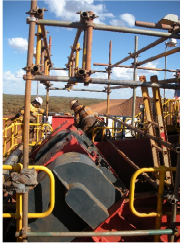
Photo No 16: Scaffolding built to provide a work platform along the excitor unit
