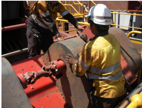
Photo No 17: Gaurds and covers being removed
