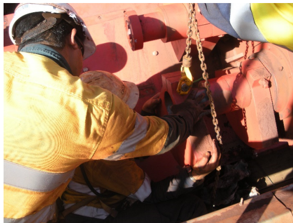
Photo No 22: Outer Counter Weight removed from keyway and shaft
