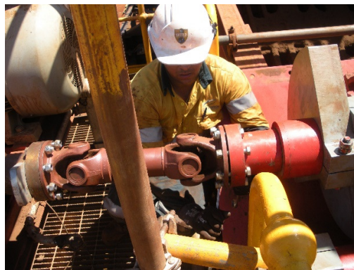
Photo No 33: Main Drive Shaft being fitted
