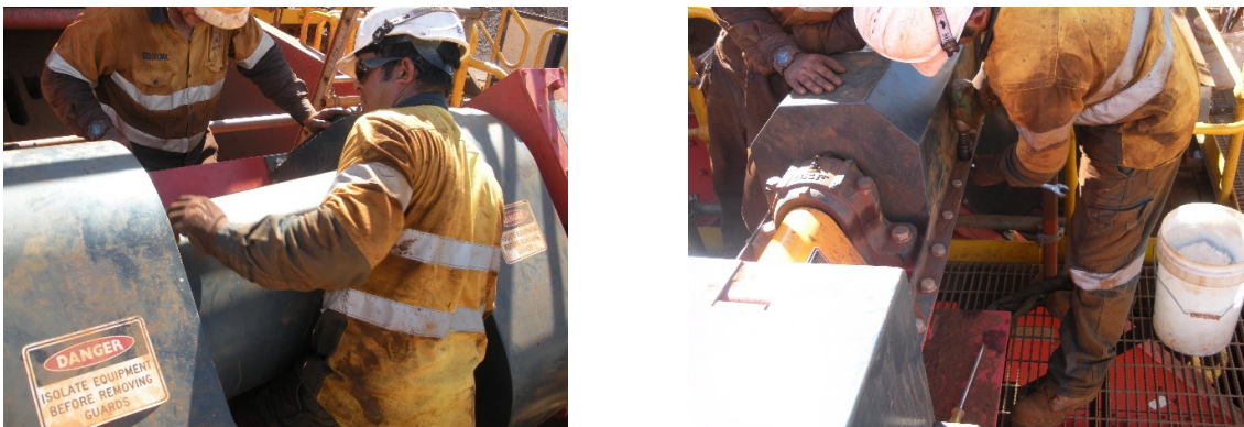
Photo Nos 35, 35A: Guards and covers re-fitted
