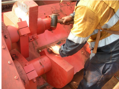
Photo No 28: Counter Weight clamping bolt lock nut being tensioned.
