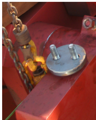
Photo No 20: Outer Counterweight locking plate removed
