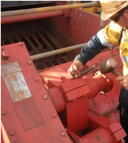
Photos No 14 and 15: Original and re-oriented position of counter weights on actuator.
