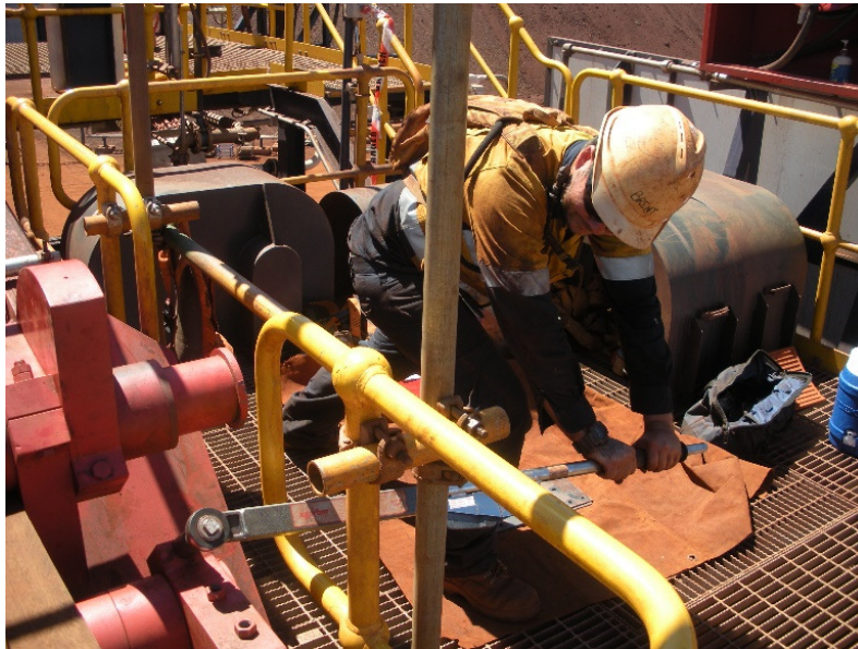
Photo No 27: Clamping bolt on Outer Counterweight being torqued.
